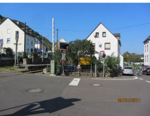
The gate crosses but one half the road; however there are two gates, both blocking the right side of the road (just like Bradley Junction on Hwy Y). Simple reflectors served to catch the motorist's eye on the gate. The warning light was mounted above the cross buck on its own post.
